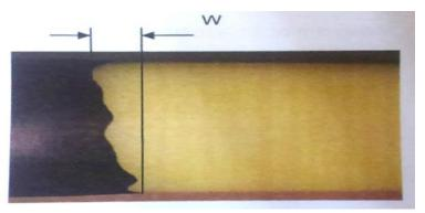
Apply a mark with insulating tape on the outer semiconductor layer in the direction to the cable so that the cable core can be peeled with the peeling device up to 10 mm before the cone. The cable core must be coated with gliding grease if the device doesn't use rolls. The round peeling device must be firmly placed at the cable end whereby the peeling knife must not rest on.
